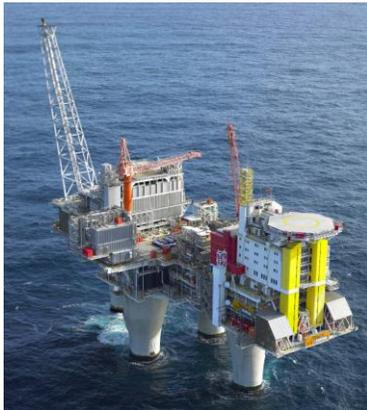
**Figure 2. Gravity Base Fixed Platform**
